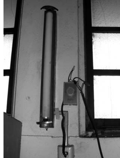
E008 - Torrance Tower, illegal wiring for exhaust fan
