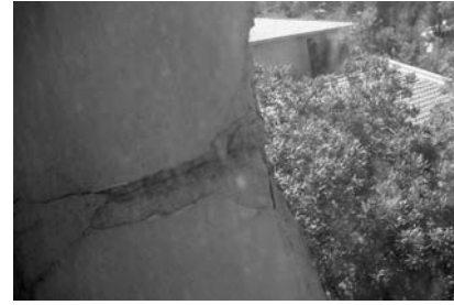
S004 - Caracol Tower - crack at window jamb
