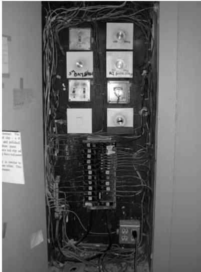
E005 - Sprague Hall panel showing multiple code violations
