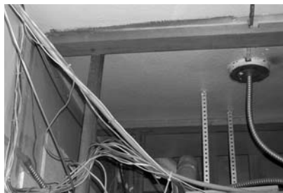
E012 - Administration area; exposed, illegal wiring condition
