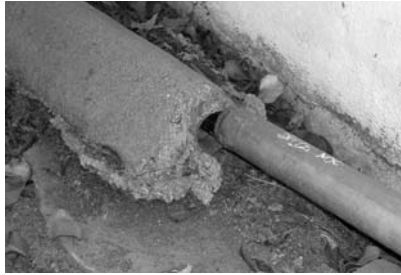
E004 - Exterior power conduit exposed to moisture
