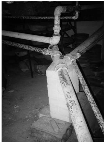
P001 - Corroded galvanized steel water pipe
