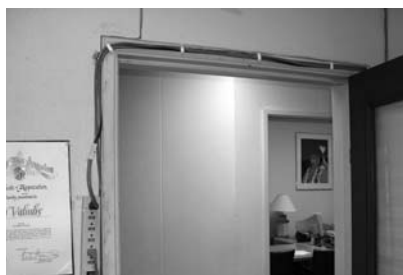
E013 - Administration area; extension cord used for permanent wiring
