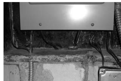
E018 - Bottom of Upper Southwest Hall panel showing illegal switch in panel cavity
