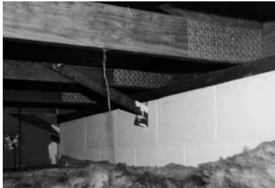
S005 - Braun Library - Connection of roofing diaphragm to wall
