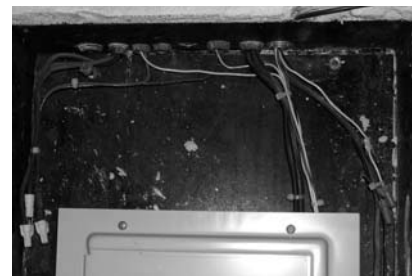
E017 - Upper Southwest Hall panel showing multiple code violations
