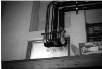
M004 - Condenser piping enters Caracol Tower through window
