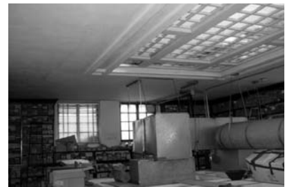
HR035 - Torrance Tower: false skylight below; historic skylight above
