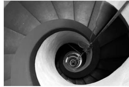
E015 - Caracol Tower stair - exposed, unsupported conduit
