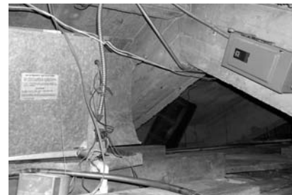
E009 - Main Building attic, illegal wiring conditions
