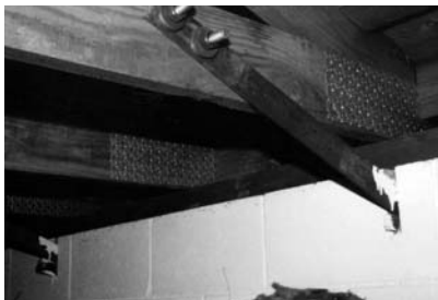
S006 - Braun Library: roof connection detail
