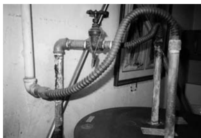
P002 - Galvanized steel water pipe; signs of corrosion
