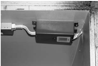
E025 - Exposed junction box and Romex connectors in display case
