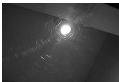
E021 - Unprotected bare display case lighting emitting UV rays; typical throughout
