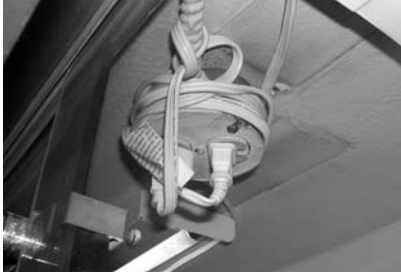
E023 - Extension cord used for permanent wiring in display case
