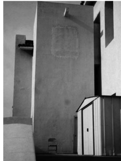
HR016 - Elevator shaft tower; east side, showing filled-in window opening
