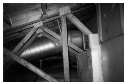
M009 - Uninsulated duct work in Braun Library
