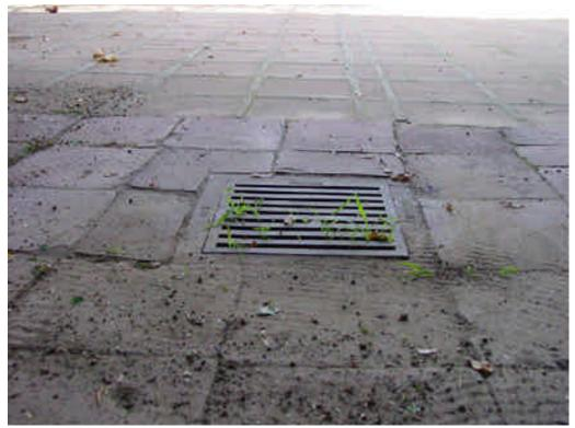
Photo 47: Drainage detail and original tile flooring at west porch area. 2005
