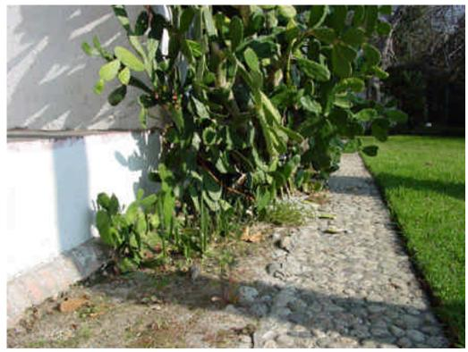
Photo 7: All landscaping should be relocated 5-10 feet away from the adobe building. The rock studded walkway is uneven and does not meet ADA requirements. 2005
