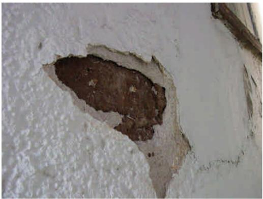
Photo 22: Detail of plaster delamination and exposed adobe. 2005
