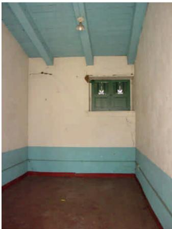
Photo 63: The Pantry currently contains nonhistoric light fixtures and exposed conduit. 2005
