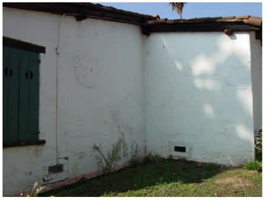
Photo 21: Northeast corner showing plaster patching, exposed conduit, and crawlspace vents. 2005
