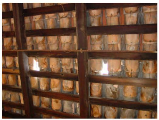
Photo 46: Missing roof tile at west porch. 2005
