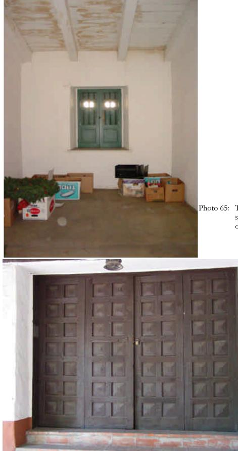
Photo 65: The Chaplain's Room shows some previous water damage on the ceiling. 2005
