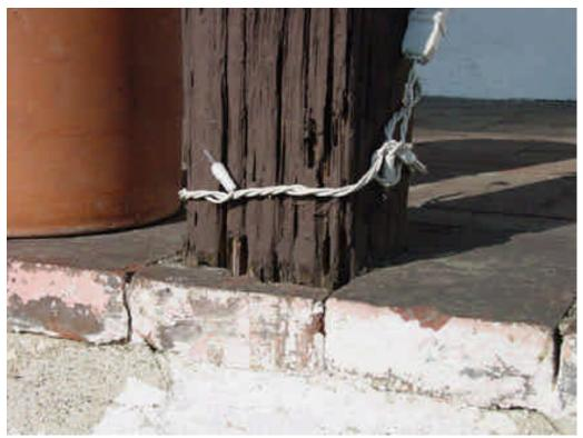
Photo 12: Dryrot at the base of the column at the entry porch. 2005
