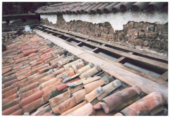
HP 27: Plaster damage and the existing tile that have been removed and drilled for seismic anchoring, 1998.
