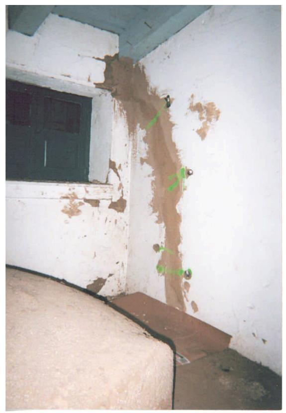
HP 23: Stitch anchoring at the northeast corner of the Horno, 1998.
