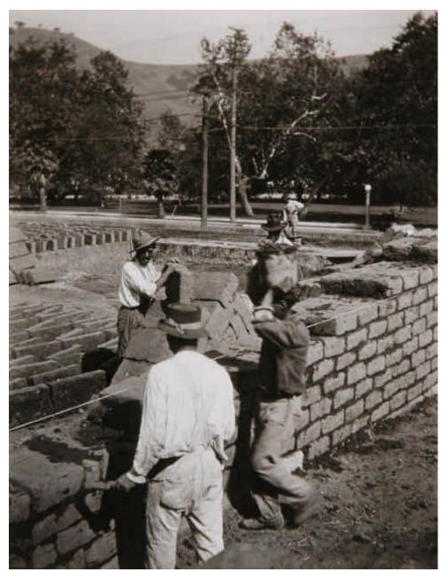
HP 2: Laying out the adobe bricks during construction of the Casa de Adobe, 1916.
