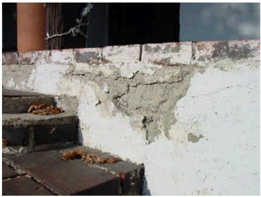
Photo 11: Plaster delamination at the entry porch base. 2005
