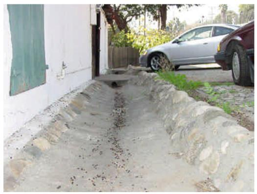
Photo 9: Original site drainage at the west elevation. 2005
