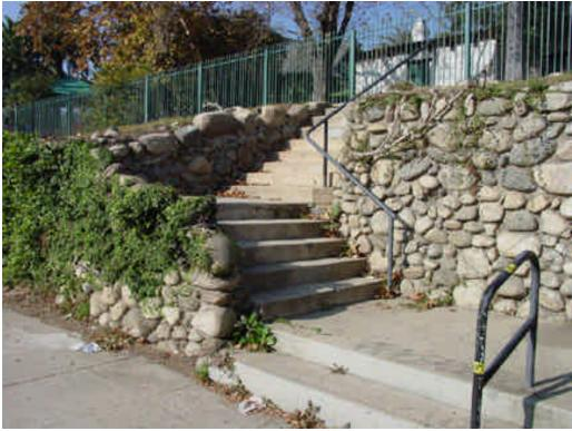
Photo 3: Street access concrete stairway. The original treads and risers have been replaced and handrails added ca. 1950s. The original risers had rock studded detailing. 2005
