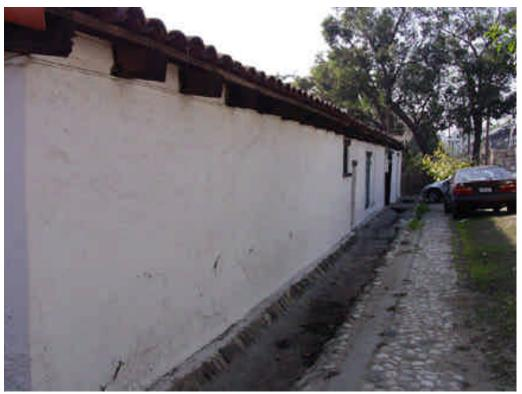
Photo 28: Plaster delamination at west façade. 2005
