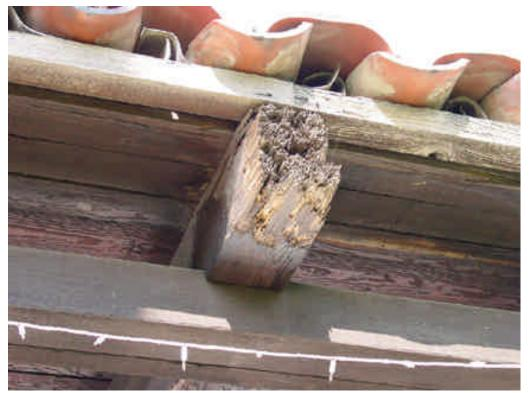
Photo 15: Rafter tail along the exterior east façade shows signs of dryrot. 2005.
