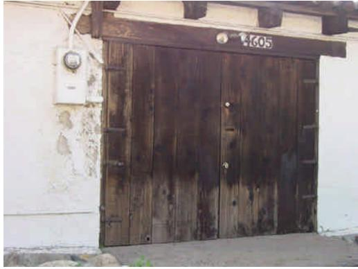
Photo 31: Original wood plank double door entry at the west façade. Note original door hardware, exposed conduit, and non-historic floodlights. 2005
