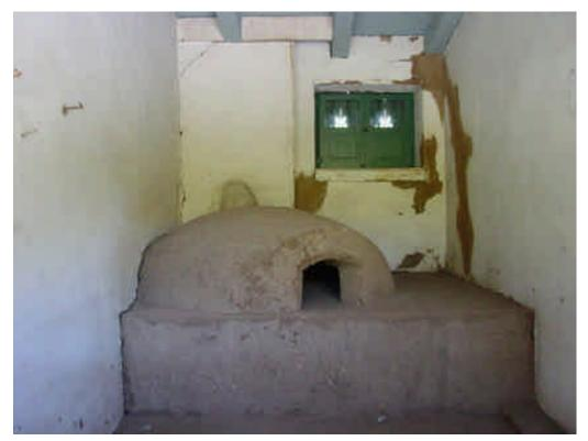
Photo 62: The Horno is unplastered. The plaster wall shows some damage at the northeast corner 2005
