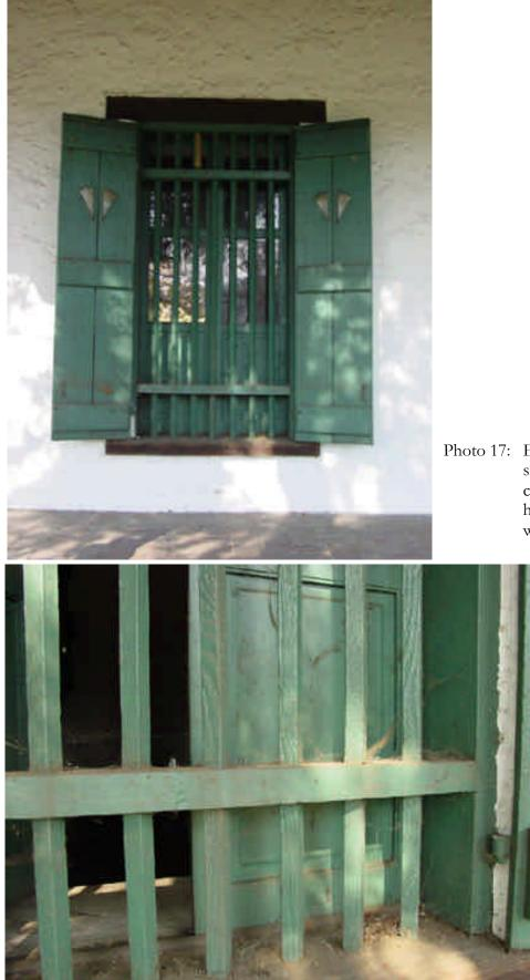
Photo 17: Exterior facing window showing wood shutter with cut out detailing, original hardware, and vertical wooden grate. 2005
