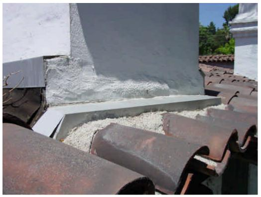
Photo 25: Horno chimney flashing detail. 2005
