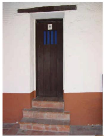
Photo 85: The original Lavatory now utilized as Men's Restroom. The restroom does not meet ADA requirements. 2005
