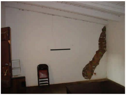
Photo 58: Dining Room looking west showing delaminated plaster and exposed adobe. 2005
