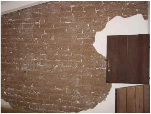
Photo 90: Delaminated plaster and exposed adobe at east wall of Children's Room. 2005
