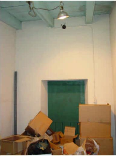
Photo 72: Museum Room showing unhistoric flood lights and exposed conduits. The east wall window is boarded up. 2005
