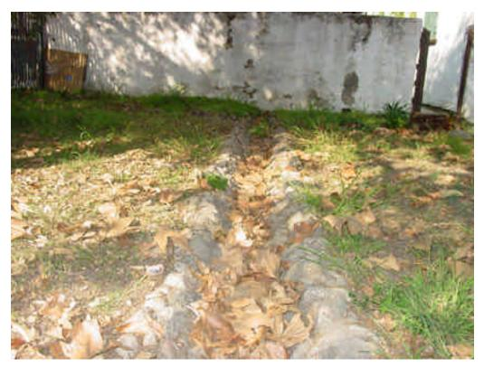
Photo 10: Site drainage at the southeast elevation needs to be cleared of all debris on a regular basis. 2005
