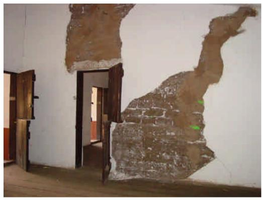
Photo 93: Sepúlveda Room looking north showing missing plaster and exposed adobe. This wall was stabilized using stitch anchoring. 2005
