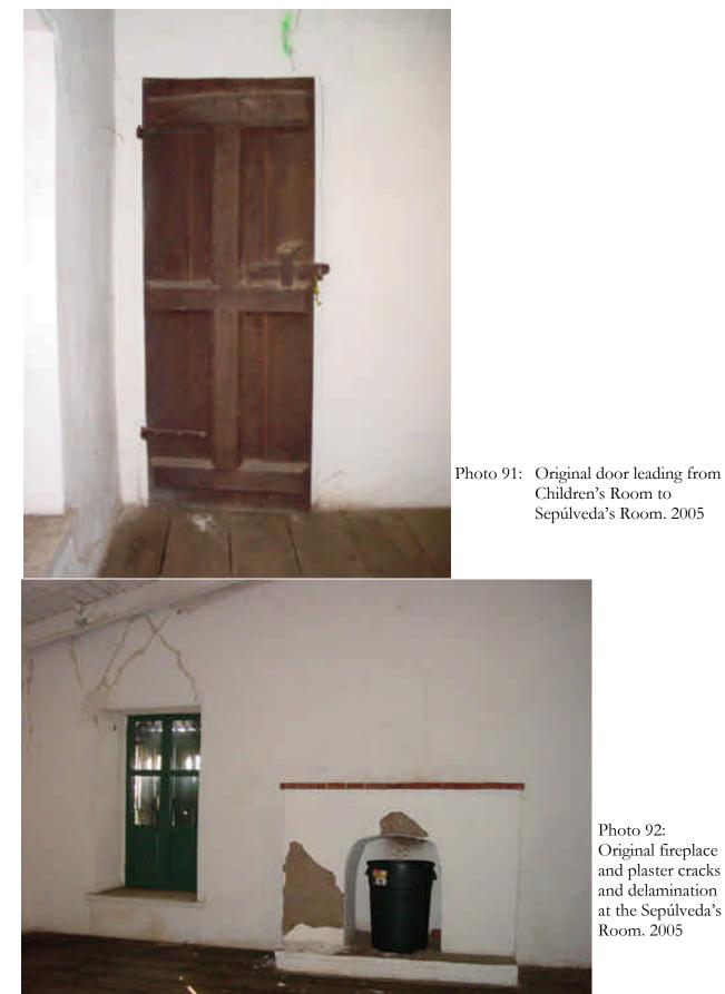
Photo 92: Original fireplace and plaster cracks and delamination at the Sepúlveda's Room. 2005
