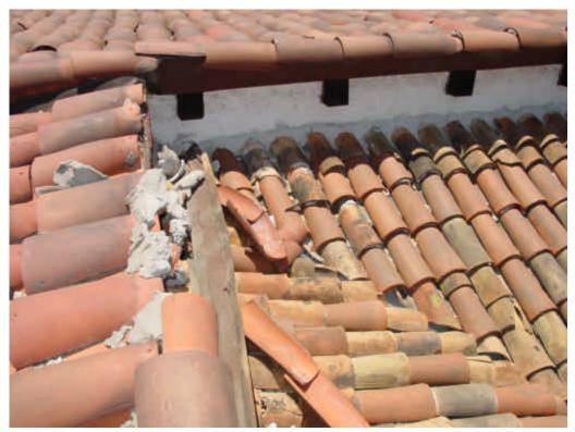
Photo 43: Northwest roof damage. 2005
