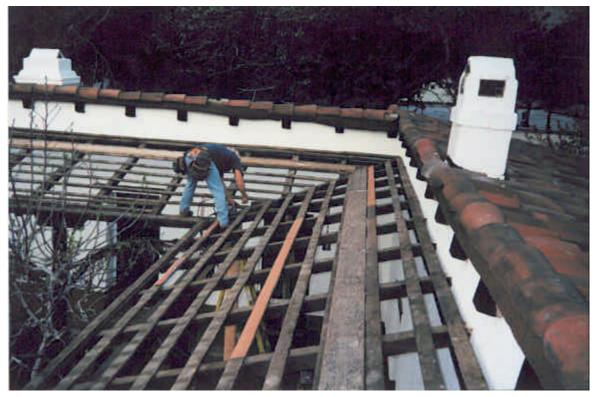
HP 26: Skip sheathing at the east porch roof as part of the 1998 stabilization project. Repointed and repainted chimney over the Kitchen at background.
