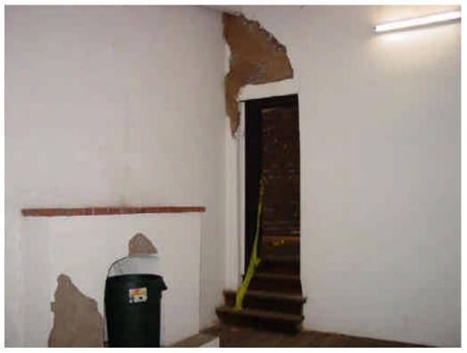
Photo 94: Doorway leading to children's room at Sepúlveda Room showing missing plaster and exposed adobe. 2005
