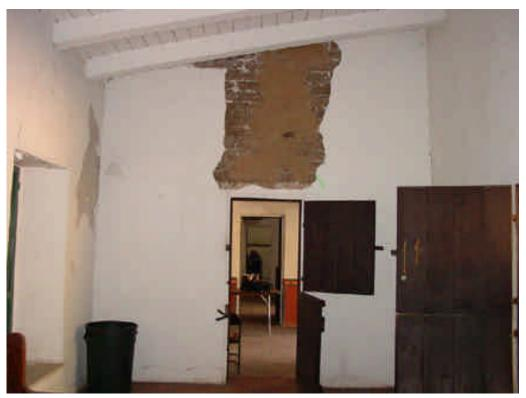
Photo 56: Looking south at Parlor showing Dutch doors and delaminated plaster with exposed adobe. 2005
