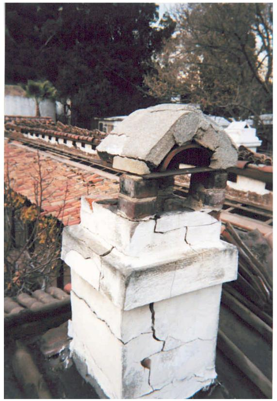
HP 25: Damage to the Kitchen chimney prior to reconstruction, 1998.
